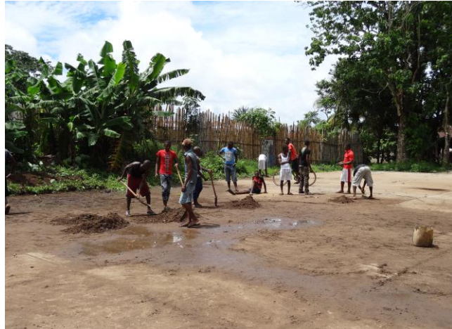
Photo – Team renovating the court
